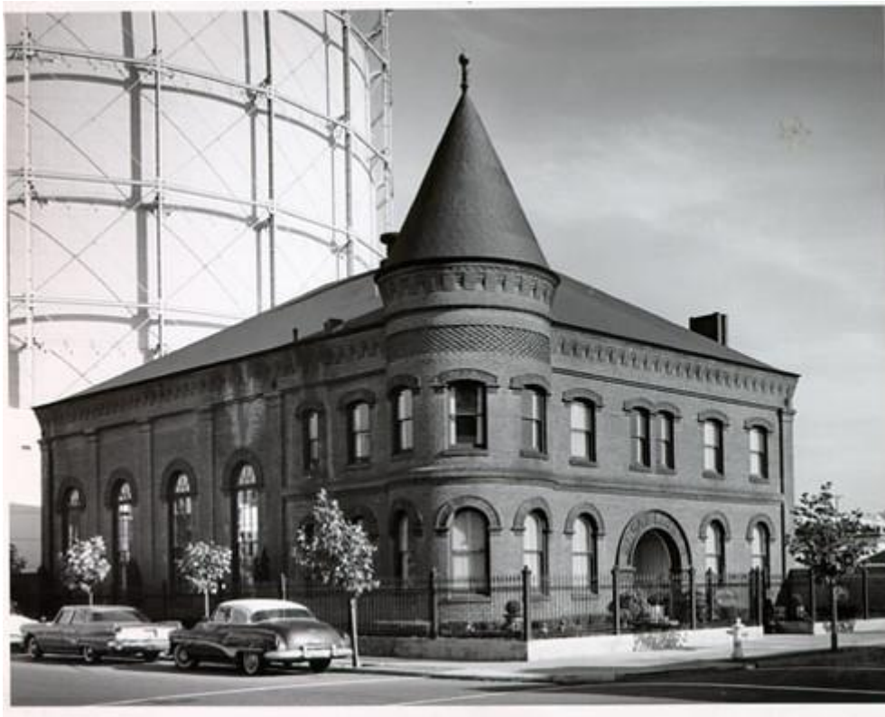
Figure 12: The San Francisco Gaslight Co. building on Buchanan Street, with one of the storage tanks in the rear. “ Gas Light building, San Francisco ” by RadioNn , CC BY-NC 2.0
